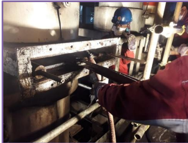
Figure 4. Repair and Installation of Mechanical Orifice After Maintenance
