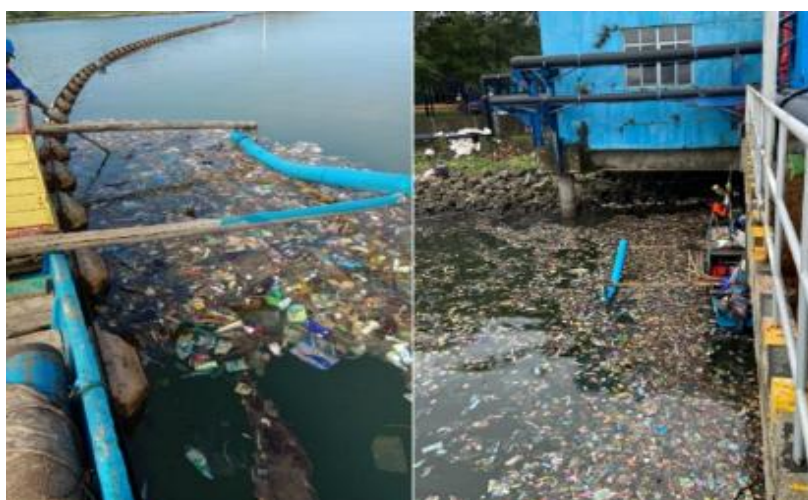
Figure. 7 Debris Accumulation at The Intake.
